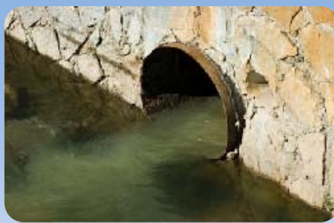
MUNICIPAL WASTE WATER
